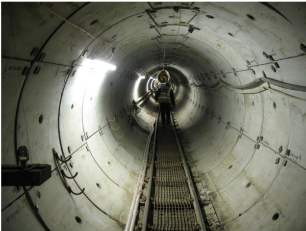
Fig. 1 Segmental lining of macrosynthetic fibre reinforced TBM tunnel
